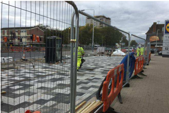
Phase 1 - Paving works underway October 2016
